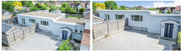
Blocked paved driveway with parking for two vehicles.
