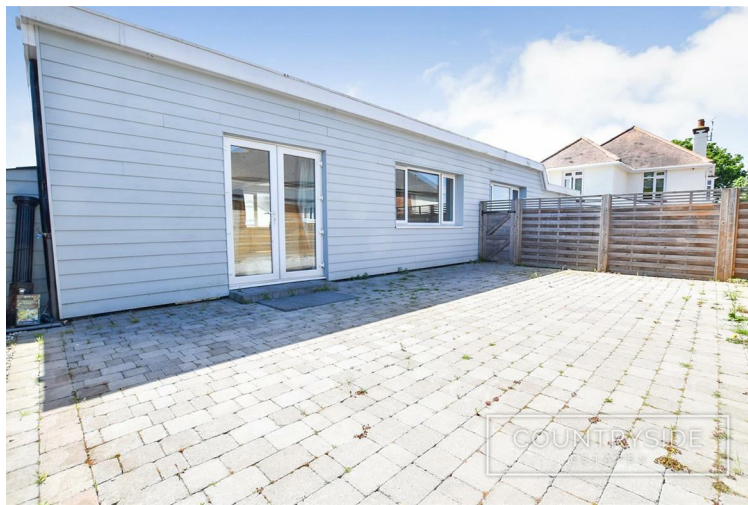
Shed 18'3" x 7'6" (5.56m x 2.29m)
